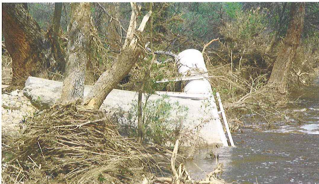
Figure 8. USGS gage in Rincon Creek, which stood for 53 years before the 2006 flood.
